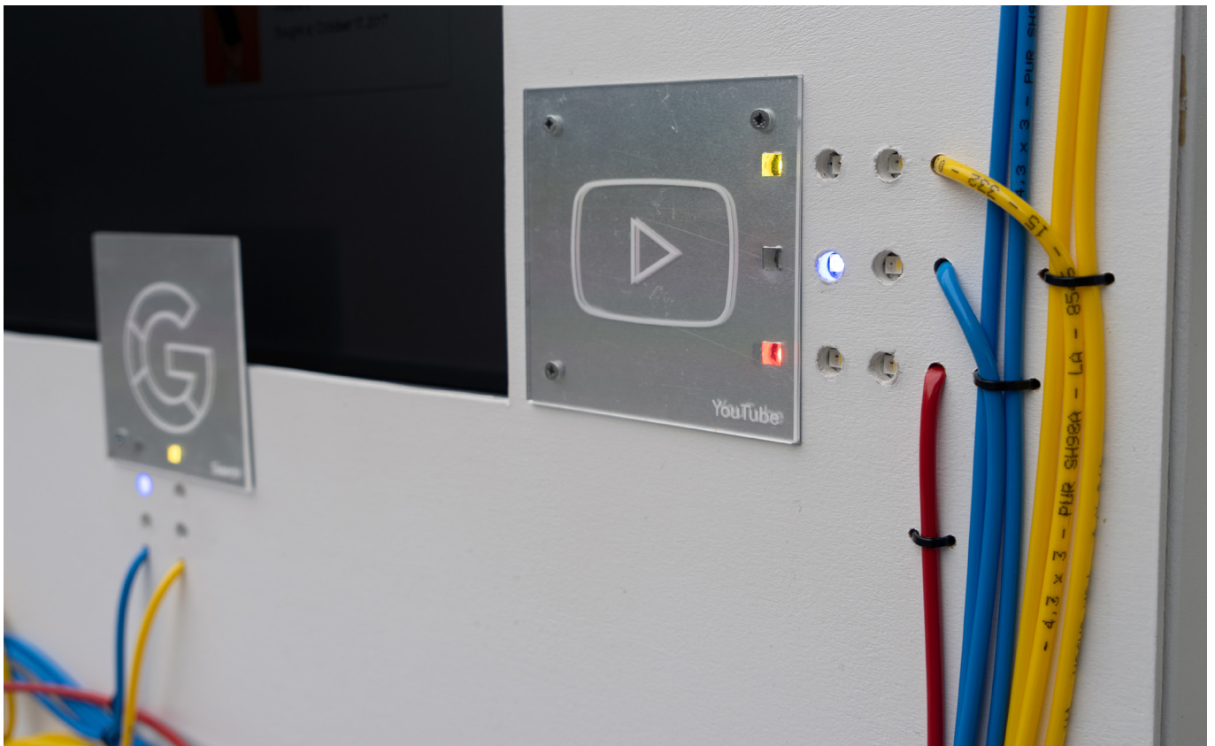
Figure 62. LEDs indicate a data stream flowing from the services into the cables.
